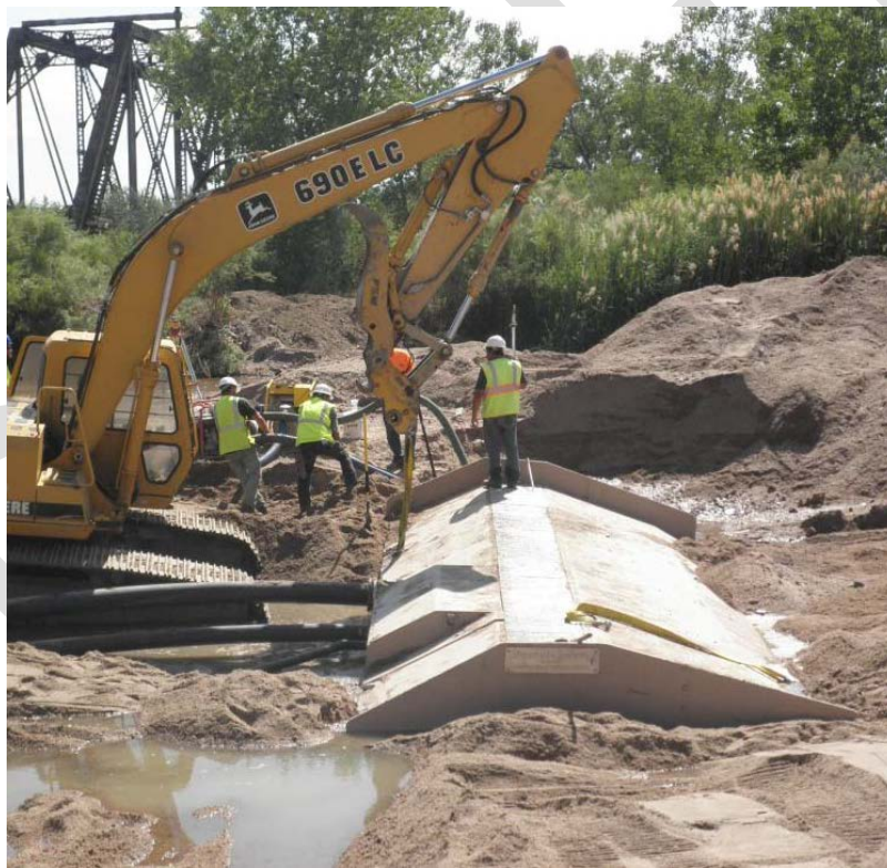
Figure 1. Installation of a 30 ft. collector.
