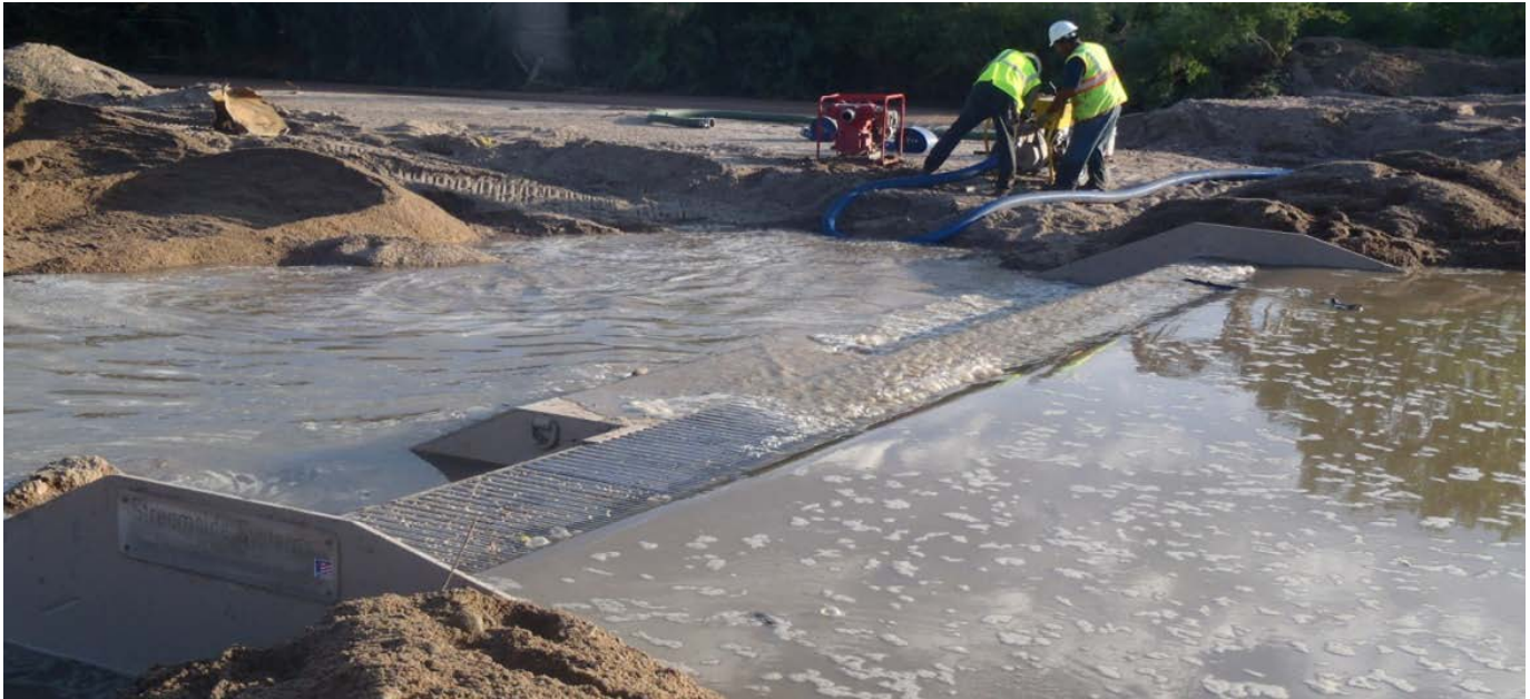
Figure 2. Sediment Collector installed in Fountain Creek, Pueblo, Colorado.
