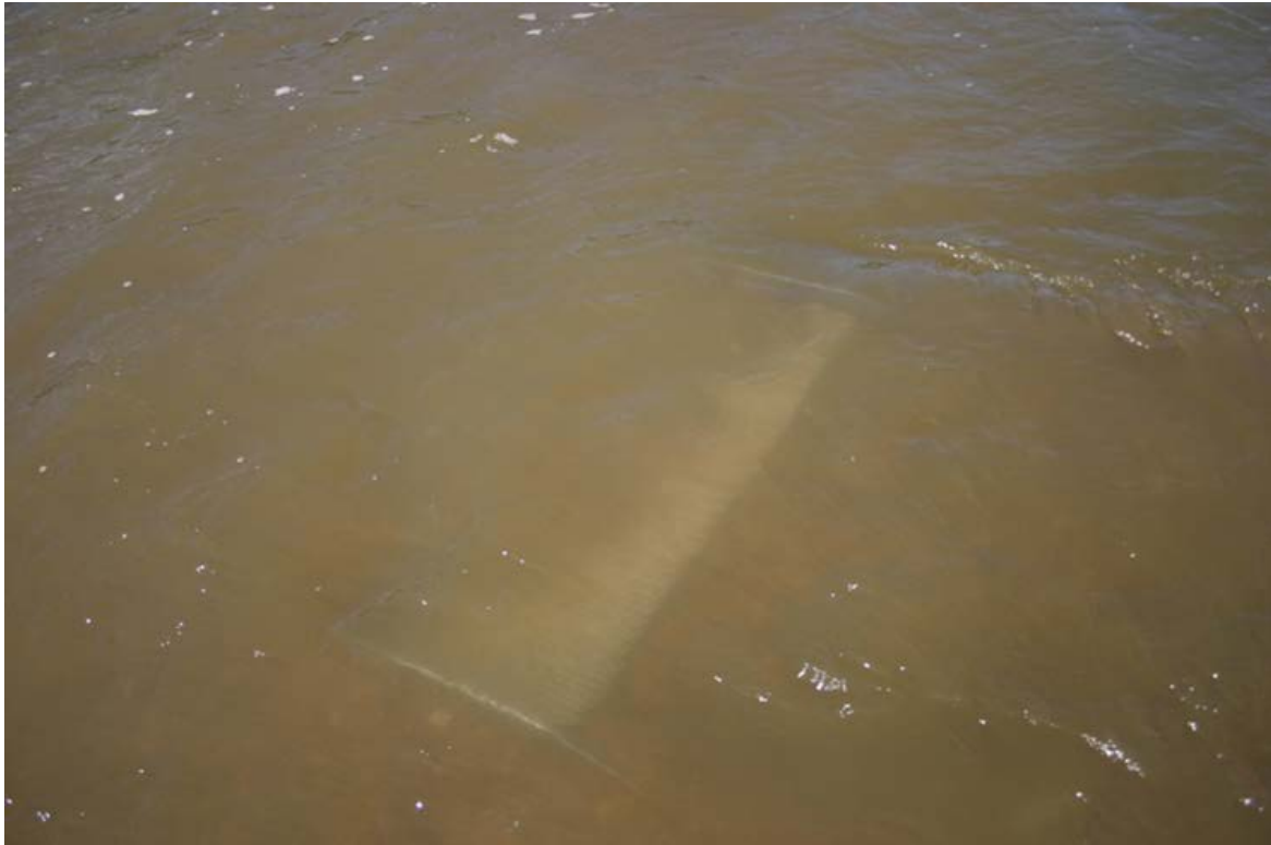
Figure 11. Gravel and sand blinding across top of 4 foot collector grate
