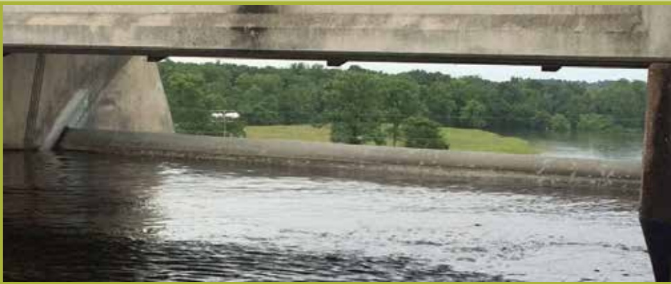
Figure 4. This photo shows the top of one of the main spillway gates at the Lake Conroe dam. At normal pool level of 201' MSL, there is approximately 18 inches of "freeboard" above the water line.
