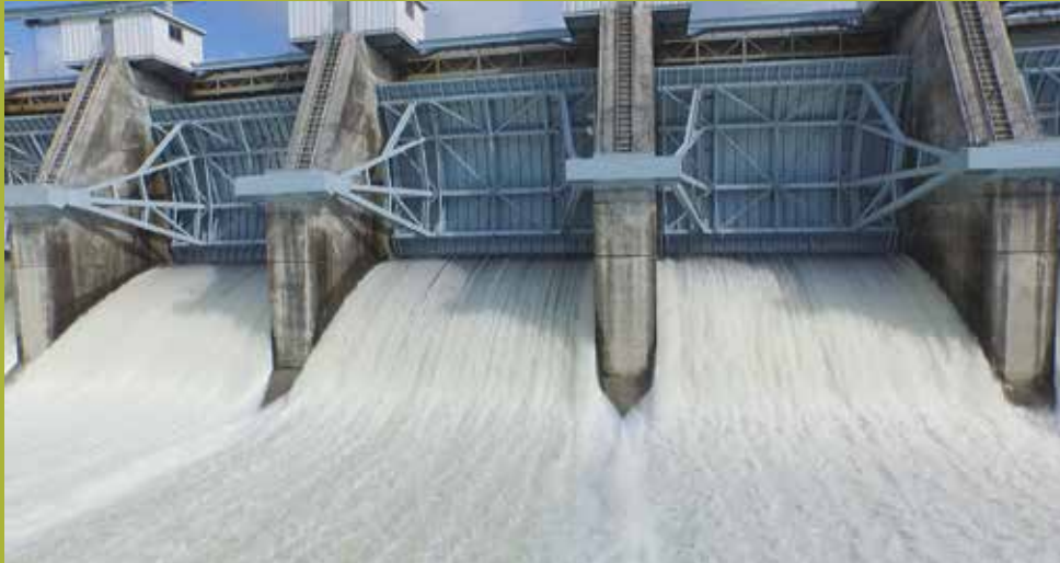
Figure 5. Back side of the main spillway gates showing storm water being released. Photo courtesy of Firefly UAV Services, LLC – www.fireflyuav.com.
